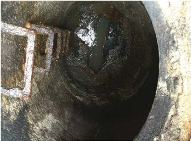
Sewer manhole before rehabilitation Photo provided by ECM Holding Group
