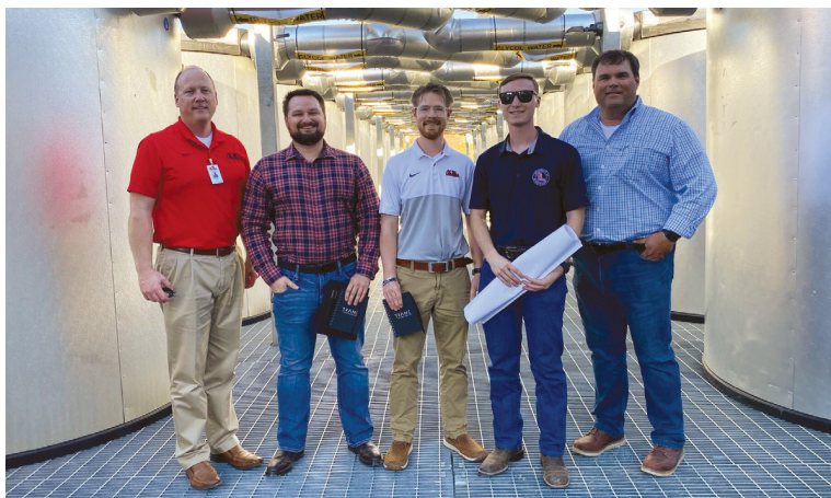
Senior Ole Miss Mechanical Engineering Capstone Group on a tour to the Mississippi State Trane Ice Storage System. Photo provided by Trane. Pictured Left to Right: Dean Hansen, P.E., Director of Facilities, University of Mississippi; Jake Shackleton, University of Mississippi student (Class of 2024); Matthew Bickerstaff, University of Mississippi student (Class of 2024); Hunter Wilson, University of Mississippi student (Class of 2024); and Chad Moore, P.E., Principal, Engineering Resource Group, Inc.
